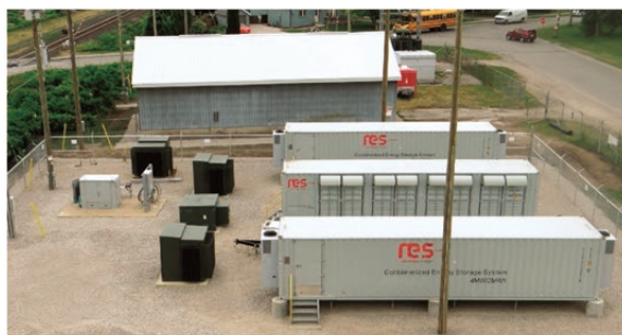
4MW/2MWh Ontario, Canada Completion time: April. 2014 Owner: RES Application: Frequency regulation
