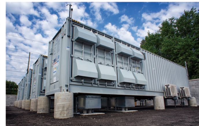
WC 19.8MW/7.865MWh ESS System Parameter Project Location: WC, USA Completion time: Dec. 2015 Owner: RES Application: Frequency regulation
